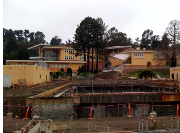
New Pool Has Walls; Mechanical Room Next
