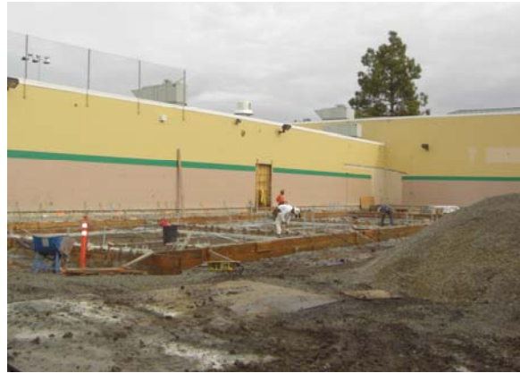
Ready to Place Concrete for Foundation
